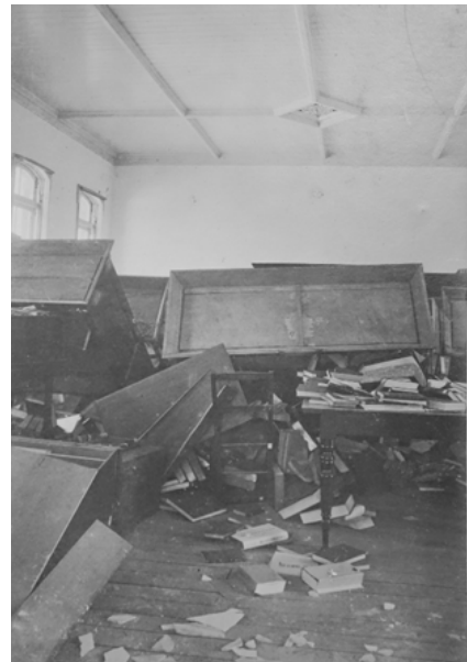
図 16 別館実験棟二階図書室本棚の倒れと散乱 Fig.16 Overturned shelf and scattered books in library in the second floor of annex building.
