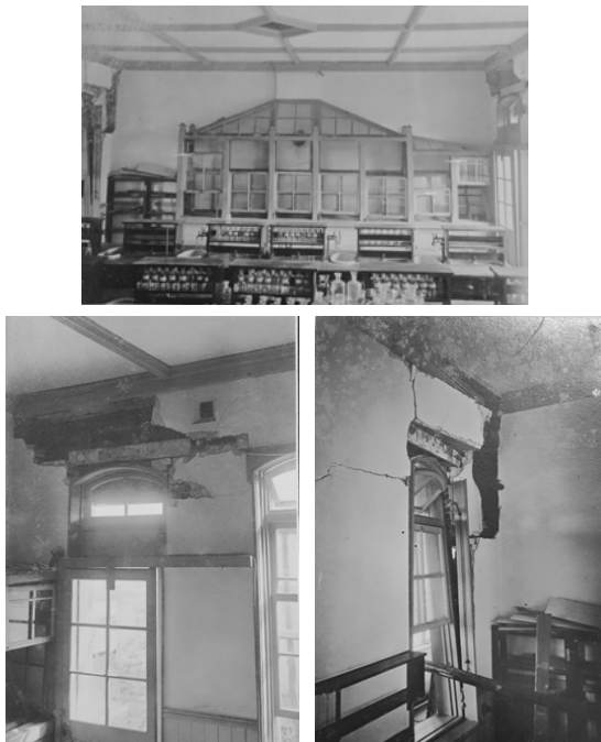
図 13 別館実験棟二階定性分析室の被害 (上:室仕切 左下:東南隅 右下:東北隅) Fig.13 Damage of qualitative analysis room in the second floor of annex building.
