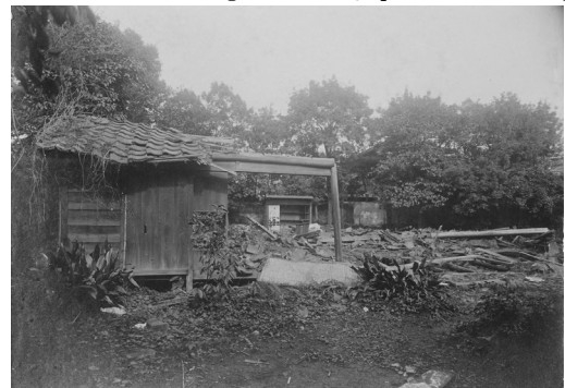
写真-5 附属官舎の倒壊 Photo-5 The collapse of affiliation official residence
